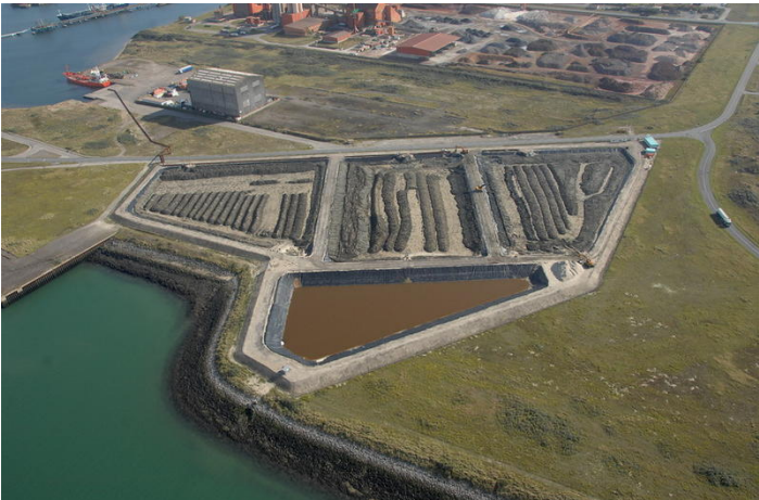
Figure 14 : Dredged treatment platform
